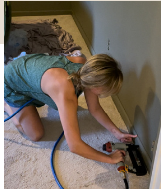
Getting dangerous with a nail gun
